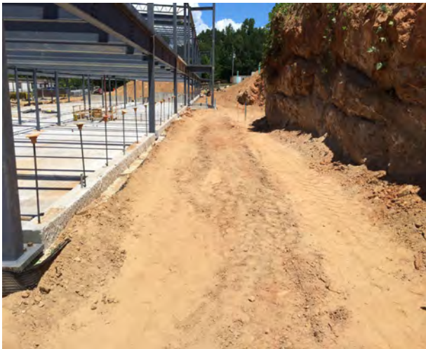
Backfilled Wall
