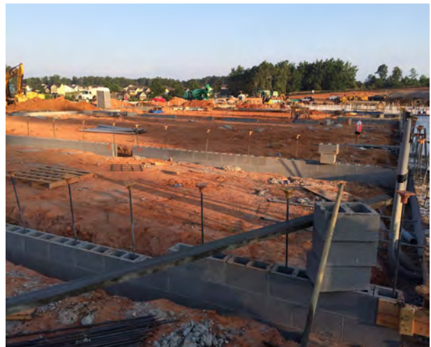
Area D Footings
