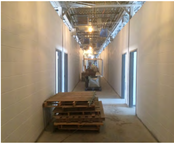
1st Floor Hallway
